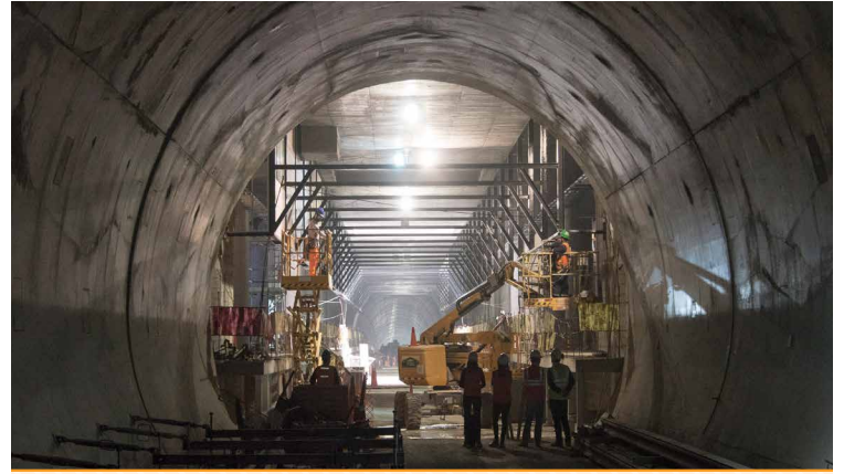
A metro line tunnel and station providing a safer and more sustainable transport system is under construction in Lima, Peru.
