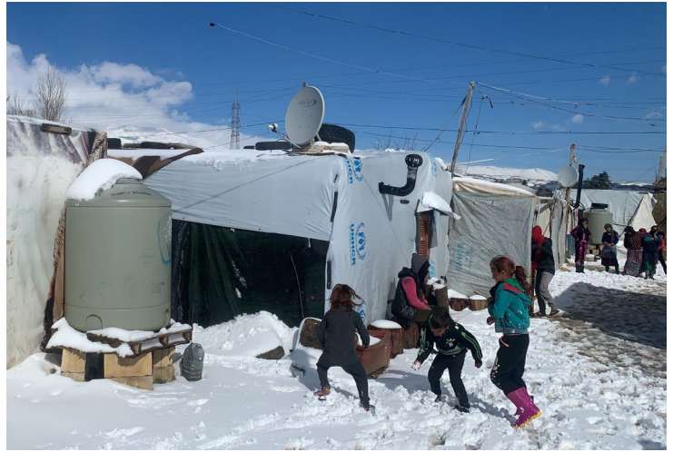
Refugees struggle after snow blankets informal settlements in Bekaa Valley. Lebanon endured one of the harshest winters in a decade in 2022. Refugees and Lebanese families struggled in sub-zero temperatures. In mid-January nearly 4,000 refugee families needed assistance. Photo: © UNHCR/Theresa Fraiha
