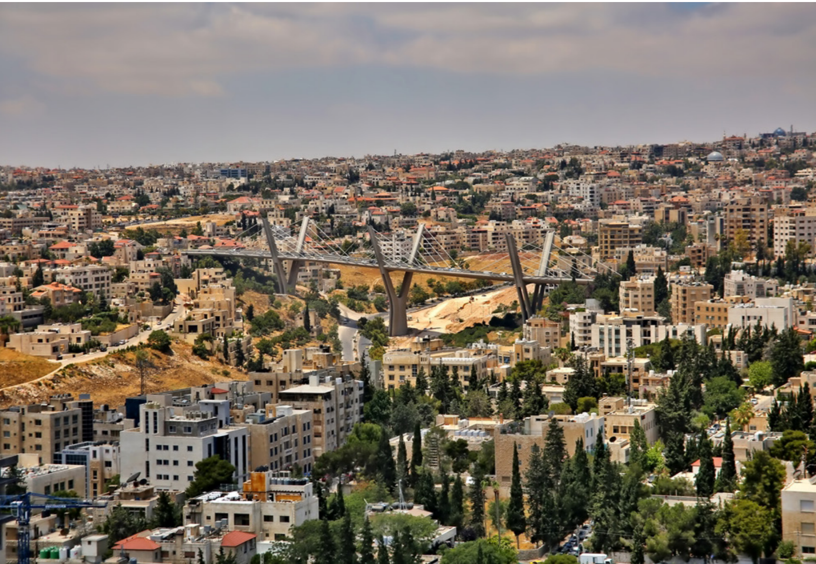
Figure 23. Abdoun Bridge, Connecting East and West Amman (Source: GAM, 2022)
