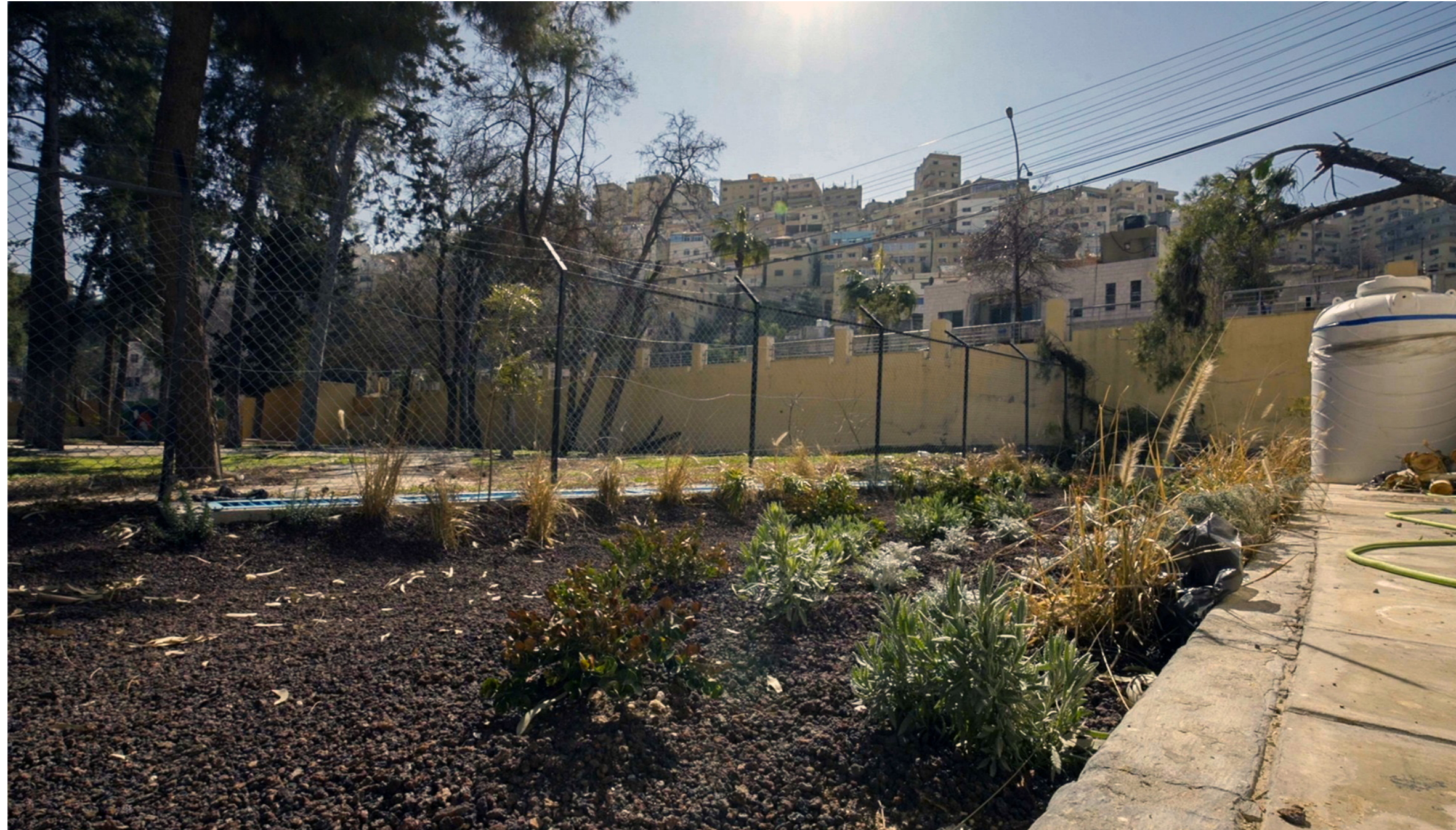
Figure 34. Rain Garden to Mitigate Flash Flood Risk in Affordable Housing Unit in Amman (Source: UN-Habitat, 2022)
