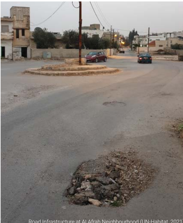
Road Infrastructure at Al Afrah Neighbourhood (UN-Habitat, 2021)
