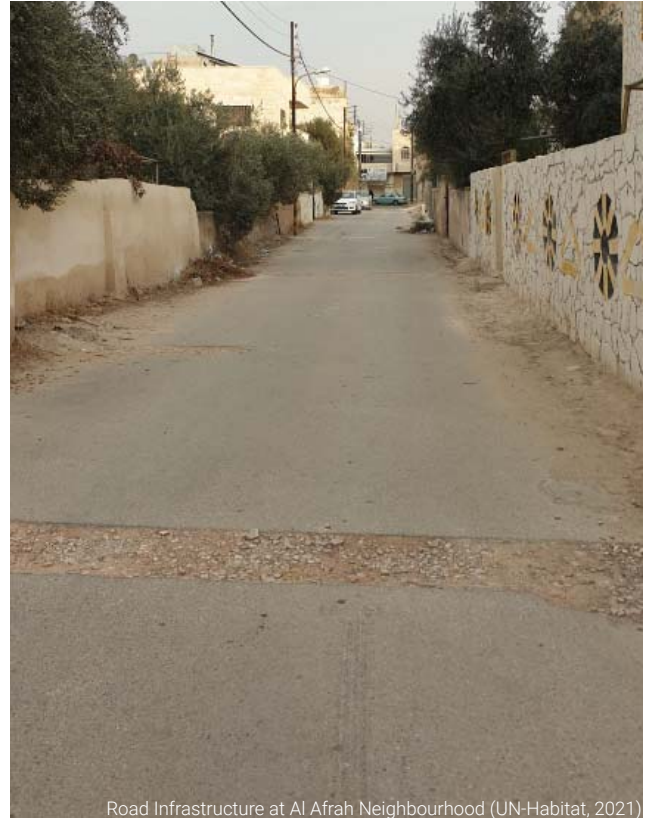
Road Infrastructure at Al Afrah Neighbourhood (UN-Habitat, 2021)
