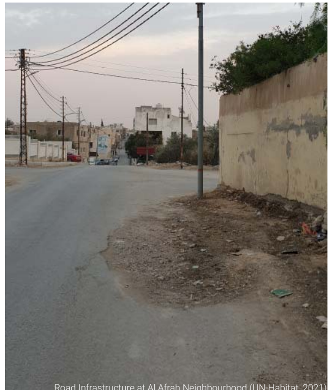
Road Infrastructure at Al Afrah Neighbourhood (UN-Habitat, 2021)
