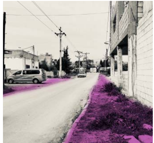
Lack of Sidewalks & Ruined Sidewalks
